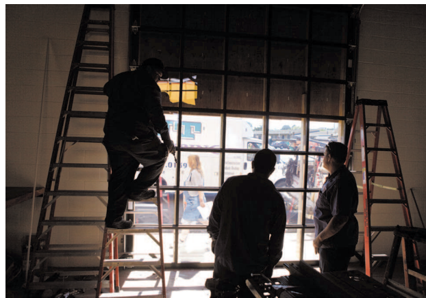
Garage door installation
