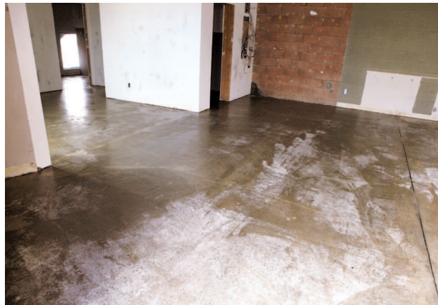
Concrete floors before sanding and refinishing
