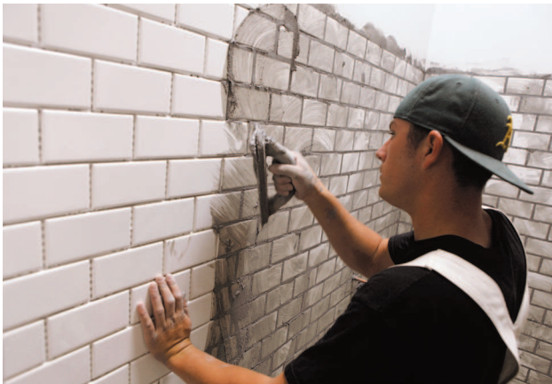
Grouting the tile — Tim Harris Tile Company
